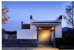
Household Energy Storage
